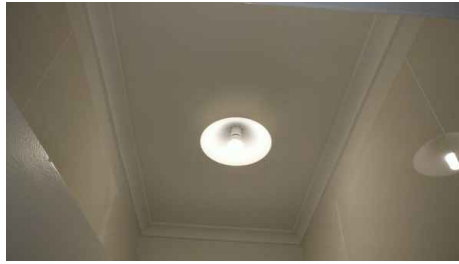
Ceiling Condition: In serviceable condition at time of inspection
