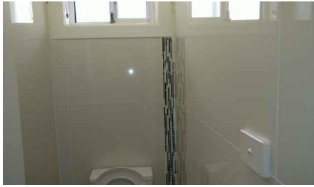
Wall Condition: In serviceable condition at time of inspection
