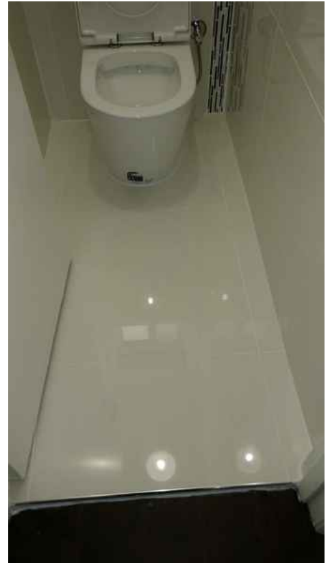
Floor Conditions: In serviceable condition at time of inspection
