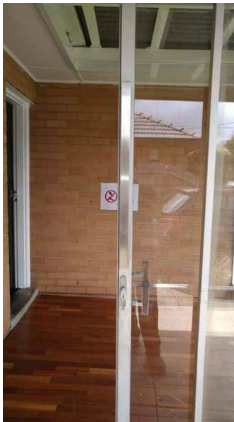
Door Conditions: In serviceable condition at time of inspection
