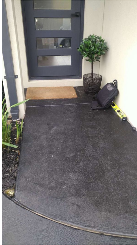
Door step/threshold: In serviceable condition at time of inspection
